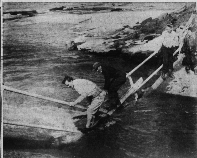
'DANGEROUS CROSSING' ONLY LINK LEFT AT ST. PETERS
