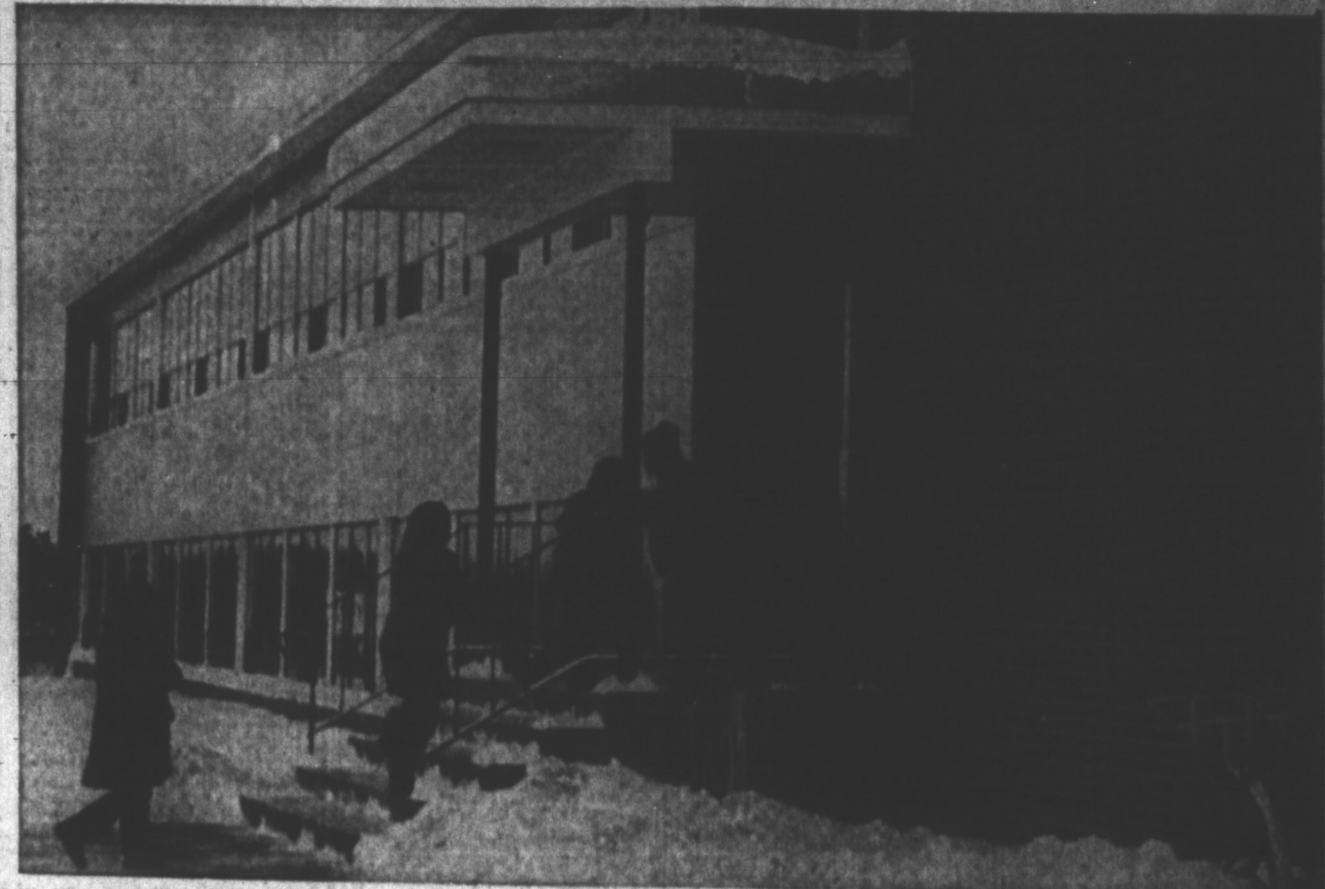
NEW 22-ROOM SCHOOL ON ELM ST REET OPENED BY PRIME MINISTER
