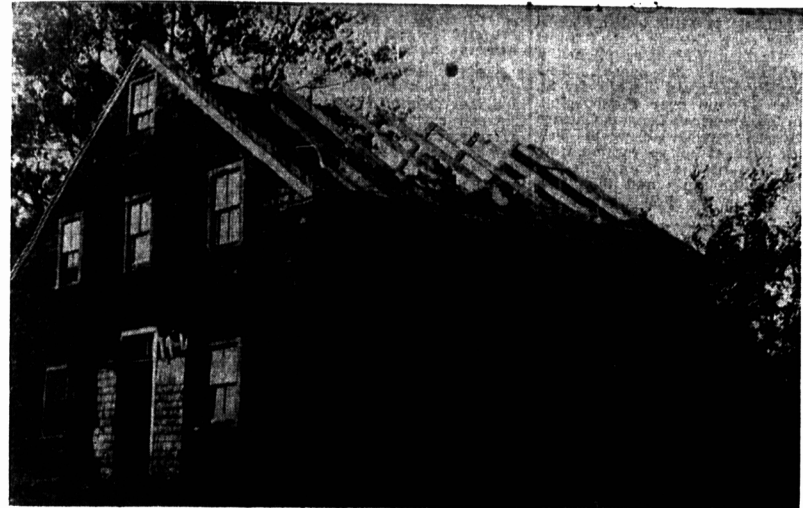
The residence of Mr. James Llewellyn, Georgetown, pictured above, lost part of its roof during the height of the storm. Debris flew across the street and broke off a telephone pole.
