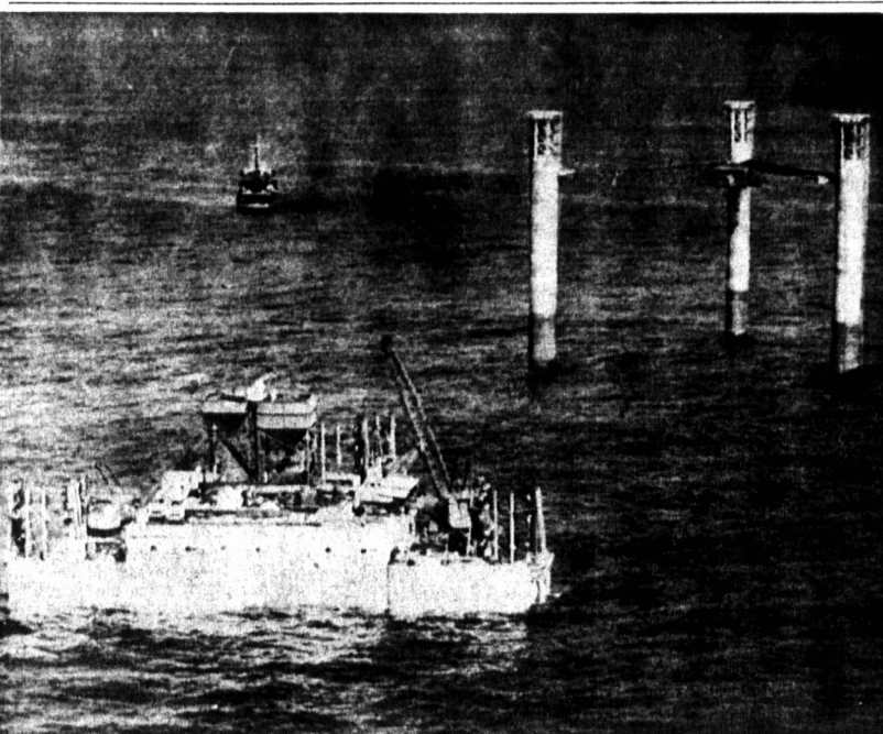
PLACING ANOTHER ISLAND The United States Government's New York City. The structure was towed from Portland, Maine, into place home 100 miles out in the Atlantic Ocean southeast of Annas, part of the aircraft warning system. It will also provide a helicopter landing spot. AP Wirephoto
