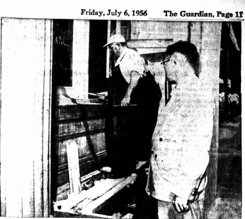
LEGITIMATE BANK "BREAK" — The Royal Bank's Charlottetown branch is not breaking into the wall so that they can install a new "Night Depository" to enable customers to make deposits outside regular banking hours.
