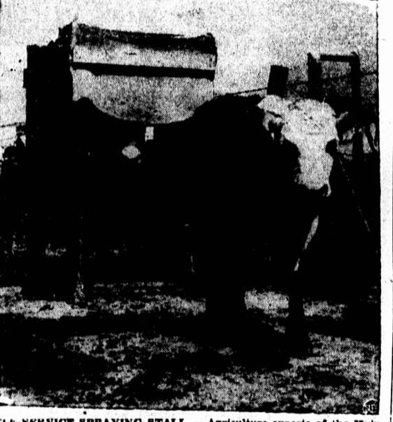
SELF-SERVICE SPRAYING STALL — Agriculture experts of the University of Illinois rigged up this bovine "beauty parlor" at Dixon Spring, Ill., where fly-tortured cattle can get relief. When Bossie walks through the stall, she trips a bellows mechanism that releases insecticide over her body, killing pesky noseflies.
