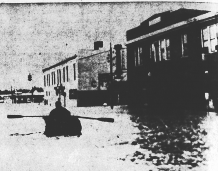
MAIN STREET BY BOAT The heart of the downtown area after the rain-washed Little River overflowed its banks. Scores of families were evacuated.
