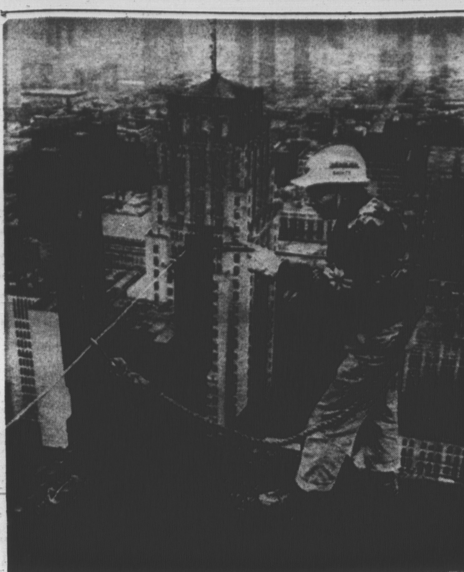
ON TOP OF TORONTO Safety supervisor Greg Doyie checks cable on the 43rd floor of the Toronto-Dominion Centre under construction in Toronto. The Canadian Imperial Bank of Commerce building is in background. When all 36 storeys are completed it will be the tallest building in Canada. (CP Wirephoto)
