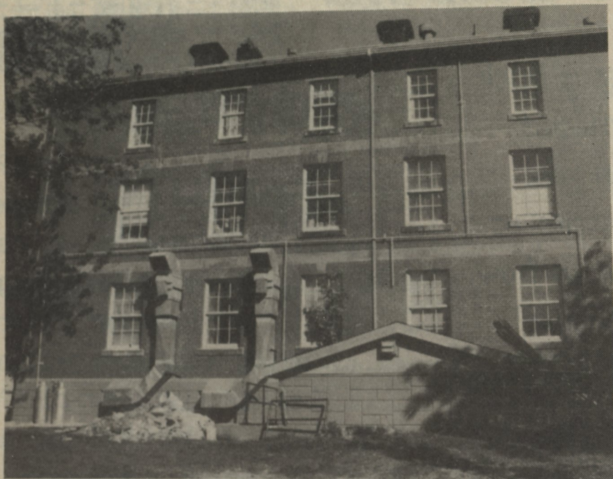
The newly rebuilt chemical shed.
