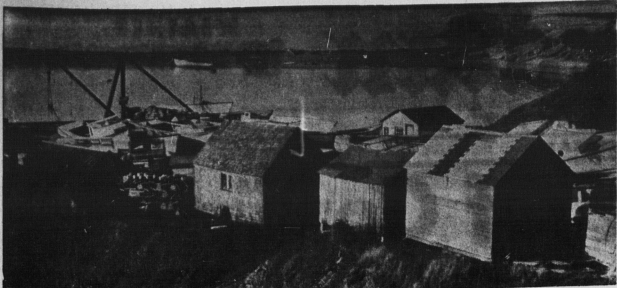
REPAIRED BUILDINGS AND ROOFS CLEARLY SEEN IN PHOTO OF HOWARD'S COVE
