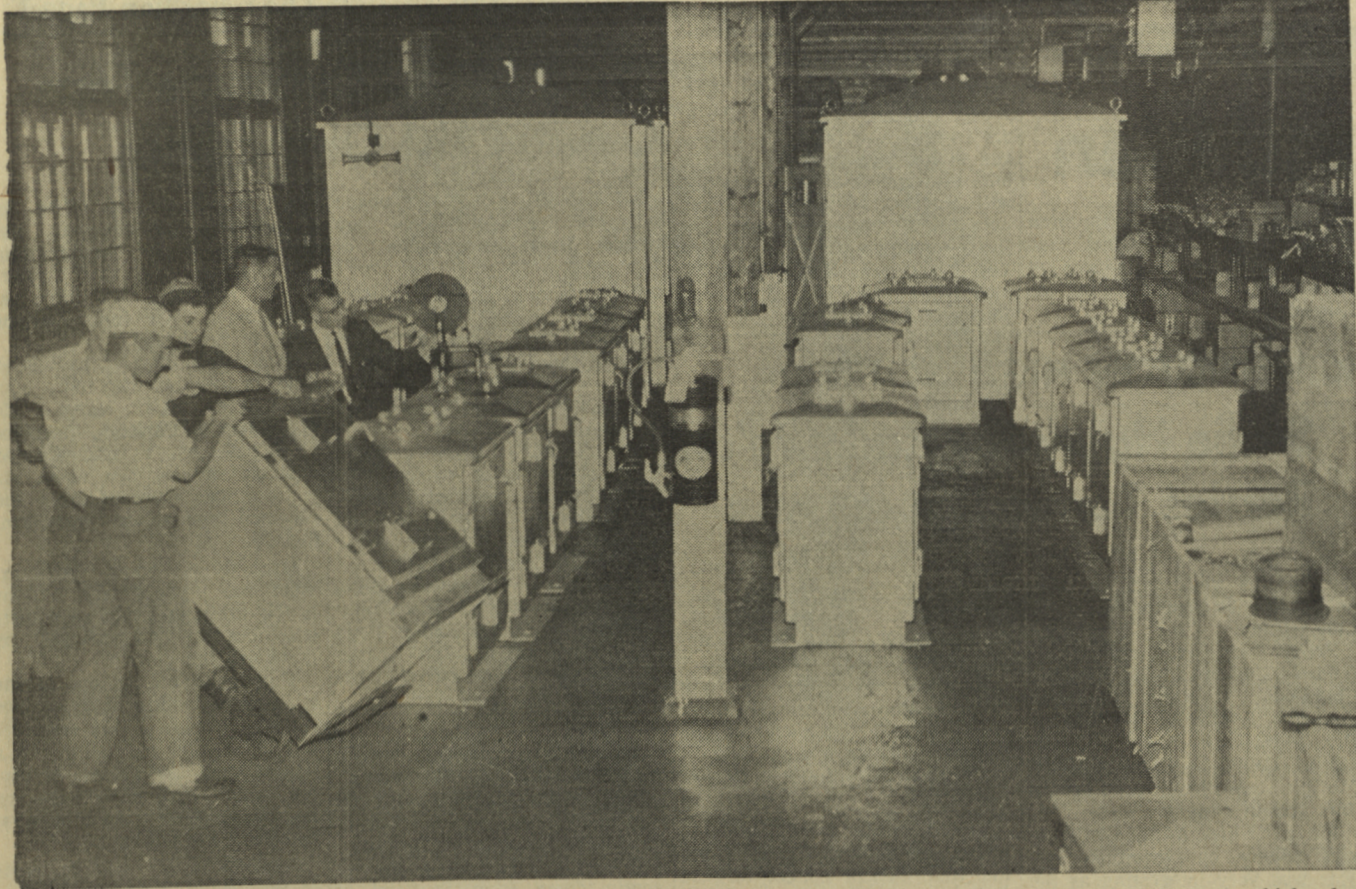
CNR SIGNALS SHOP in Moncton houses centralized traffic control equipment being prepared for shipment to installation points. At right foreground are shown stepper units crated and ready to go. Shelves behind them are laden with assembly parts. Heavy steel cases to be processed before installation line the floor. At left, one of the cases is being lowered carefully by
