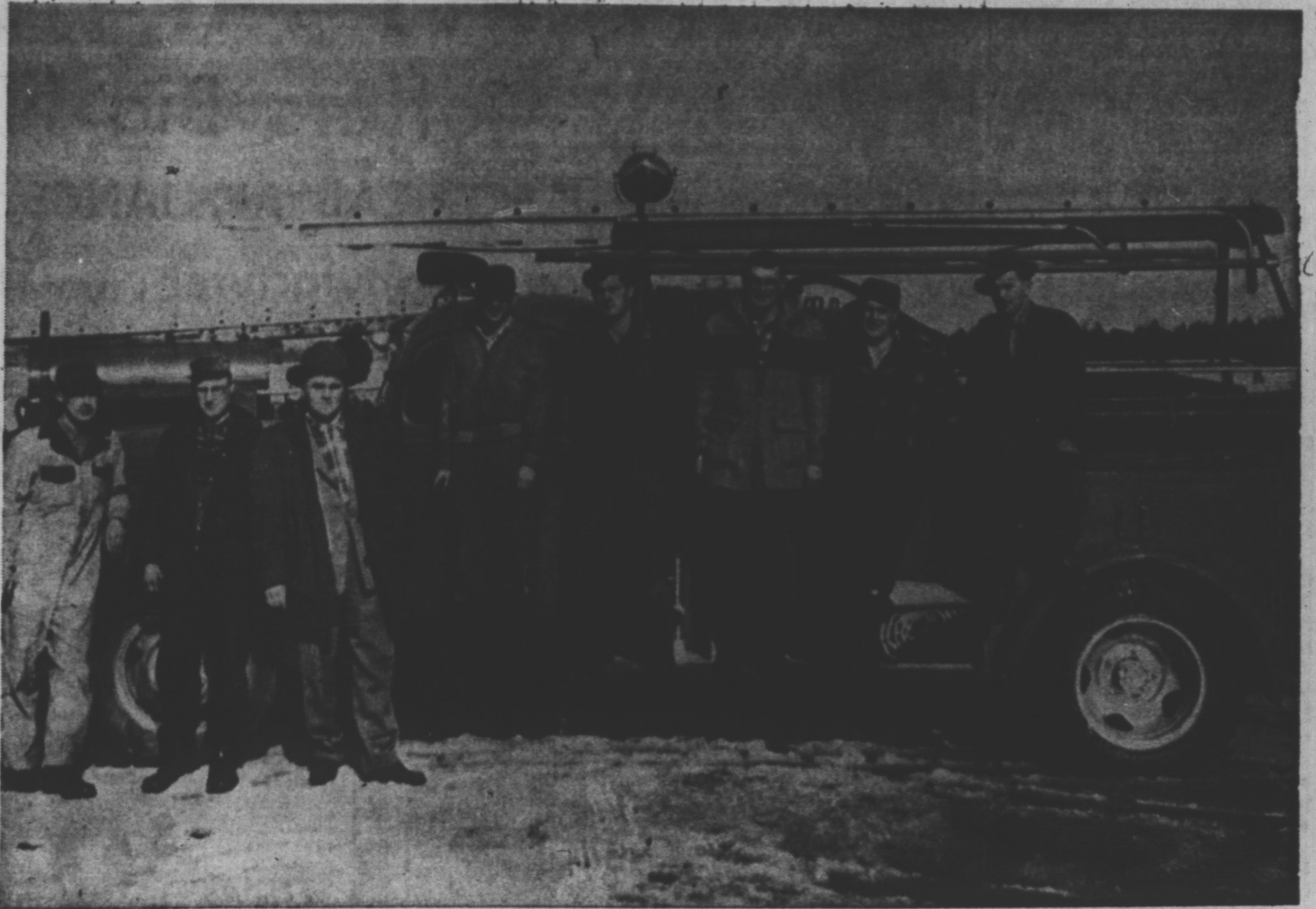
FIREMEN HOLD TEST
