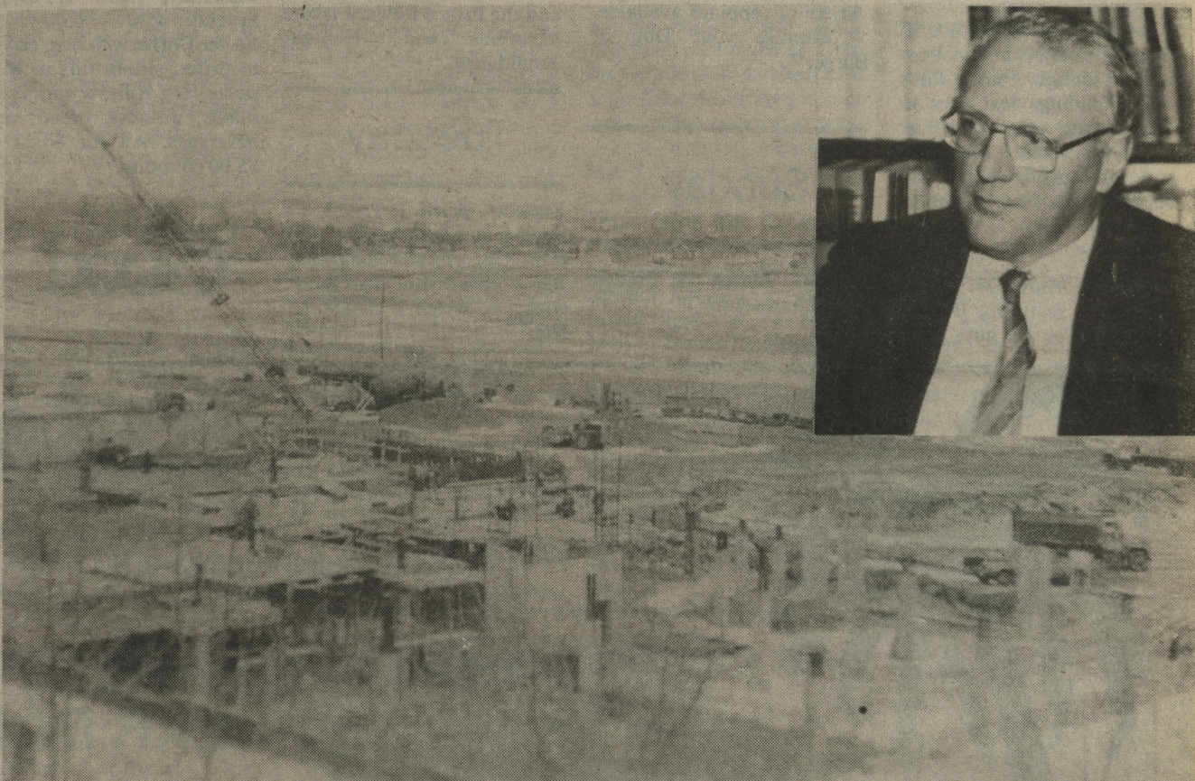
Site of the Vet College construction. Inset, President Peter Meincke, who was in power during critical negotiations for the facility. (Photos: MacLeod)
