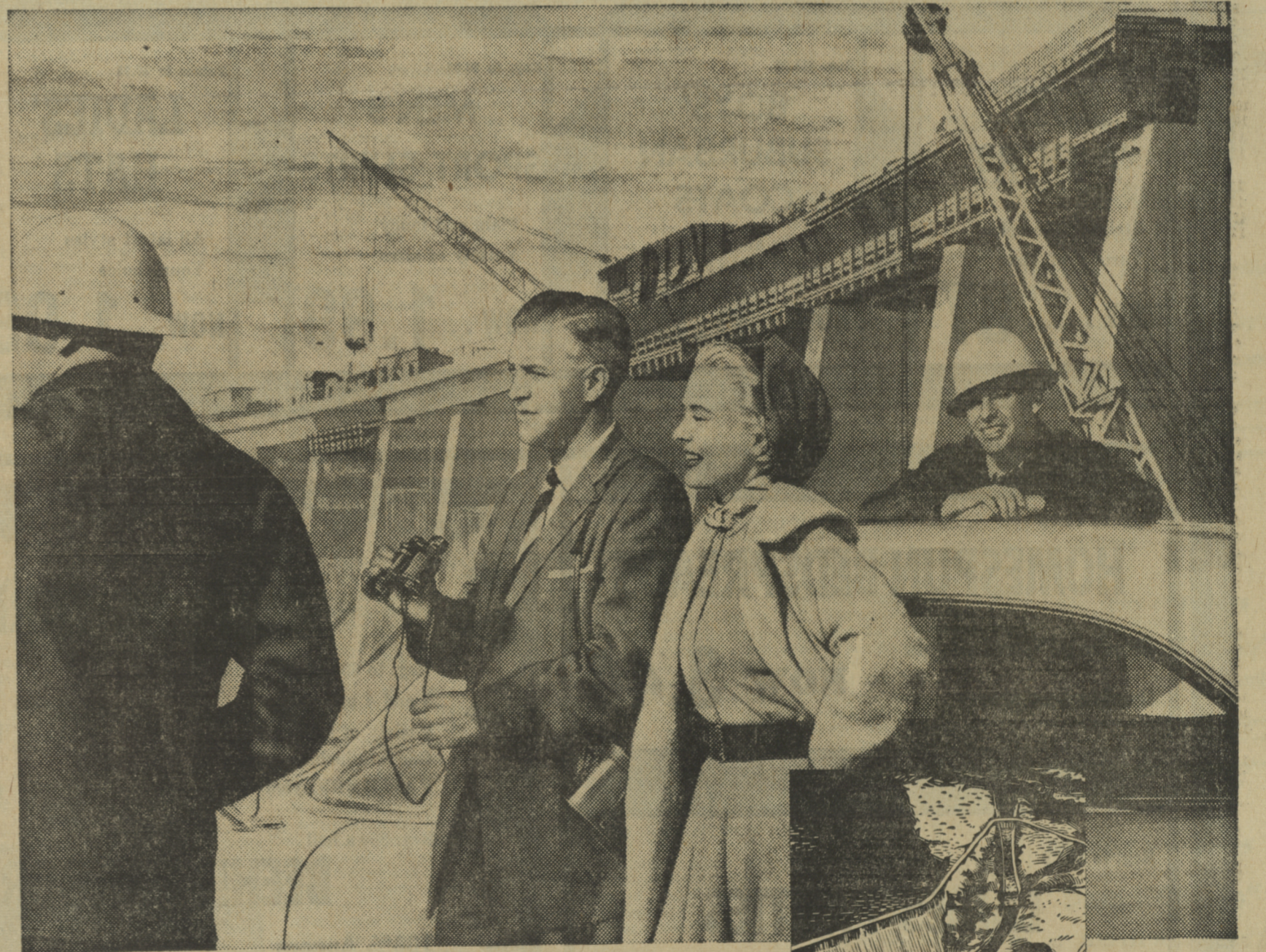
South Saskatchewan Dam (Now under construction)
