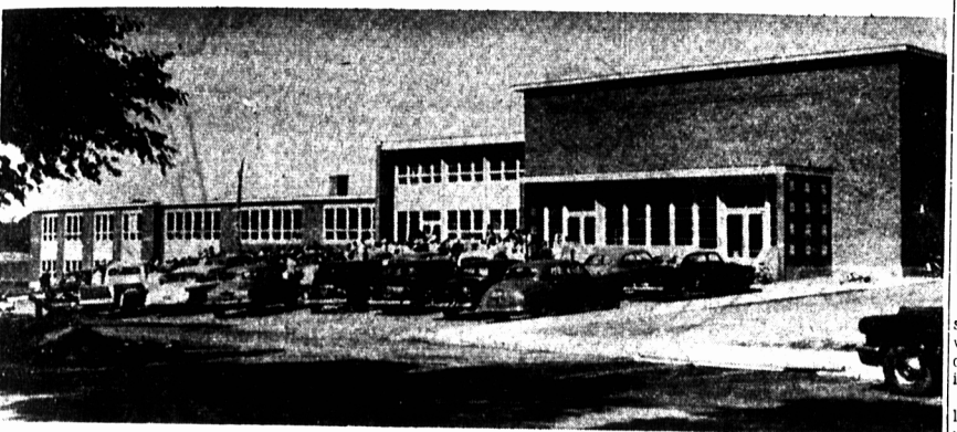
In the top picture, laying the corner-stone yesterday at the new Queen Charlotte High School. Left to right, stone mason on project, Dr. R. G. Lea, chairman of the Charlottetown School Board, Mr. W. W. Downie architect and seated, Hon. Keir Clark, Minister of Education. Below is a view of the school.
