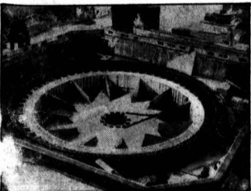
The G-E generators for the Canadian section will be built at the Company's Peterborough Works. Larger than the one being assembled, above, they will be among the biggest in size ever made. The rotating part of each generator alone will weigh over 300 tons.
