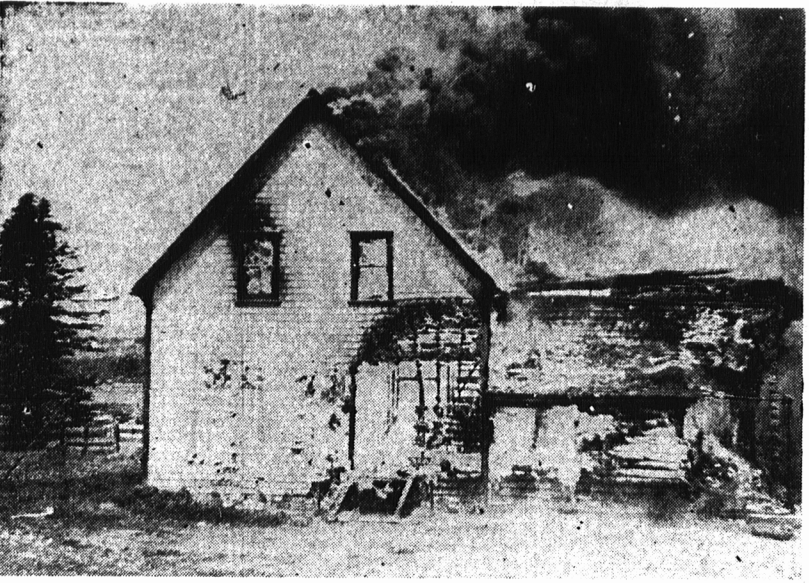
The above picture was taken during the fire on Sunday which destroyed the dwelling of Mr. Joseph S. Kelly at Fort Augustus. The loss was estimated at between $6,000 and $7,000. Firemen from Charlottetown responded to a call for assistance and helped save nearby barns.
