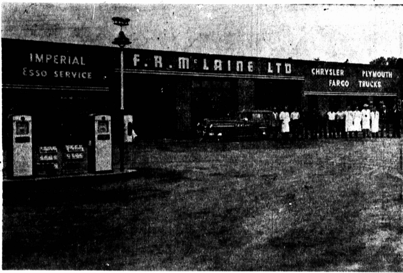
The F. R. McLaine Ltd., Service Station, Garage, Showroom, Parts and Accessories Department and Offices located on the Malpeque Road.
