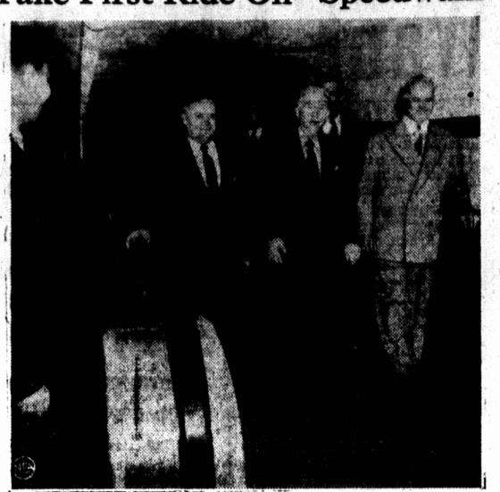
The new one-piece passenger conveyor belt at the Jersey City, N. J., tube station of the Hudson and Manhattan Railroad is put into operation. The Goodyear Rubber Company belt can carry 10,000 passengers an hour up a 227-foot-long, 10-degree rise, ramp. Riding the belt are (left to right): Jersey City Mayor Bernard J. Berry; William Reid, president of the H & M; and E. J. Thomas, president of Goodyear. This is the first such equipment to be operated in the United States.—(NEA Telephoto).
