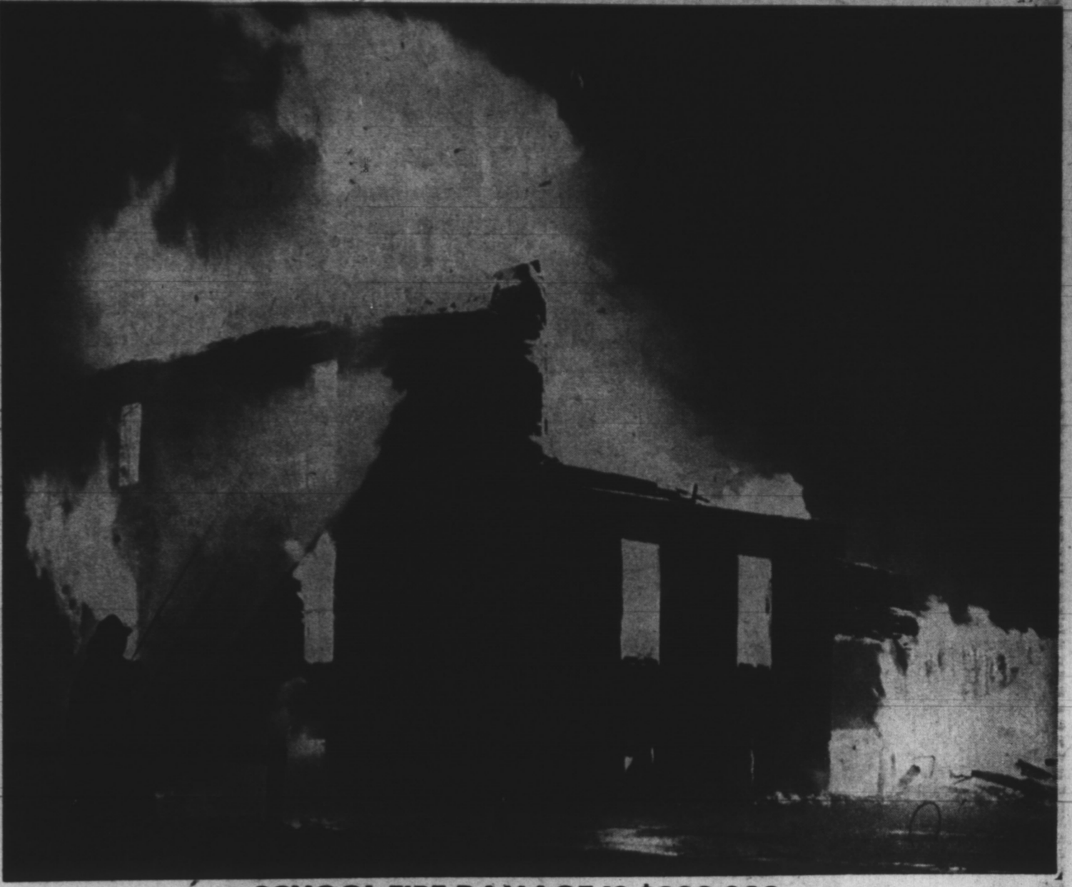
SCHOOL FIRE DAMAGE IS $300,000
