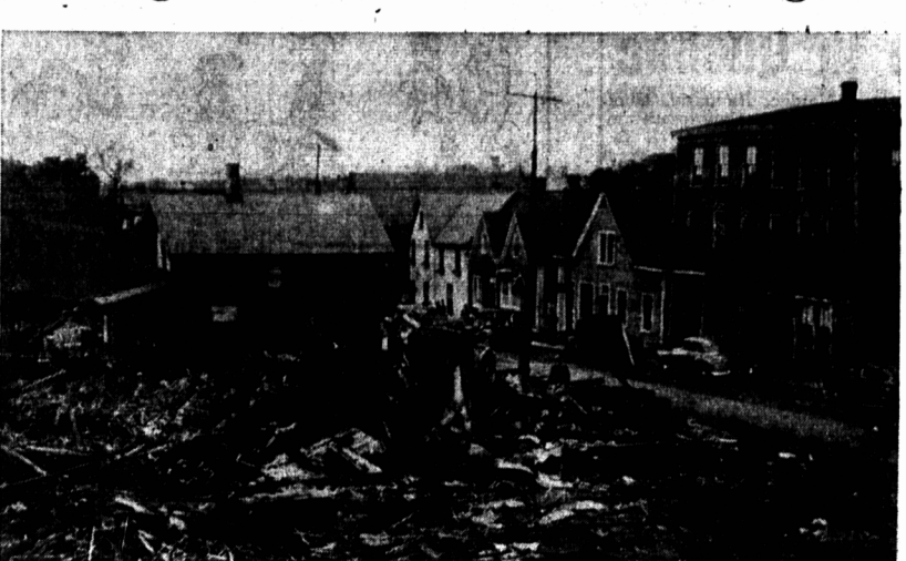
Above is part of the site of the new Federal Building in Charlottetown where demolition of present buildings has been underway for several days. The picture is looking westward from the Queen Street side along Richmond Street. The small house still intact may be moved to a new site.
