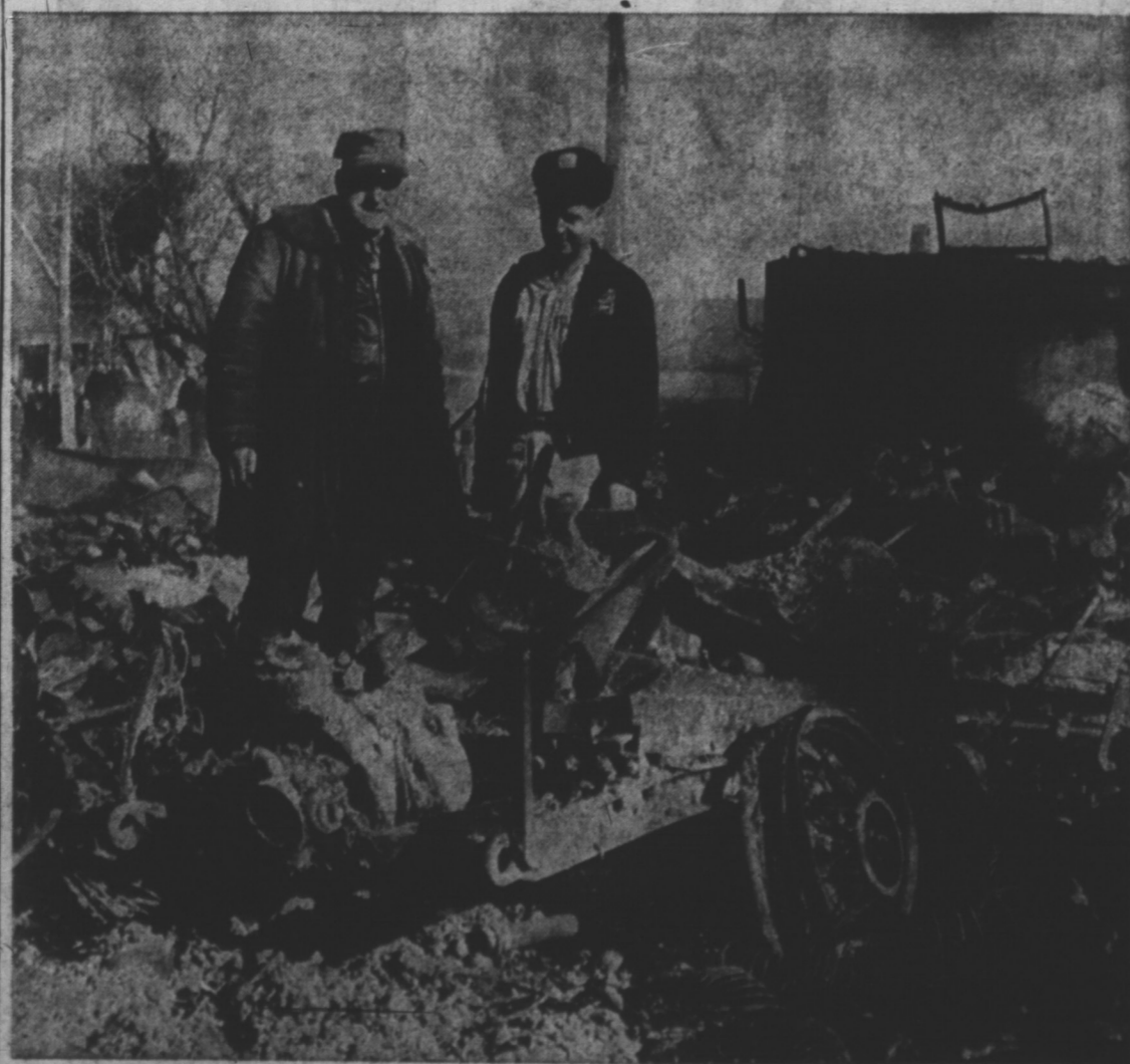
MAYOR WENDELL R. Birt, left, and Fire Chief Edmond C. Lavis take a long, sad look at the ruins of what was their fire engine. They are probably thinking of how much damage they could have prevented had the pump been in action instead of falling a victim to the blaze.
