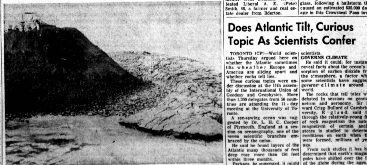
GOOD PROGRESS ON BRIDGE APPROACH
