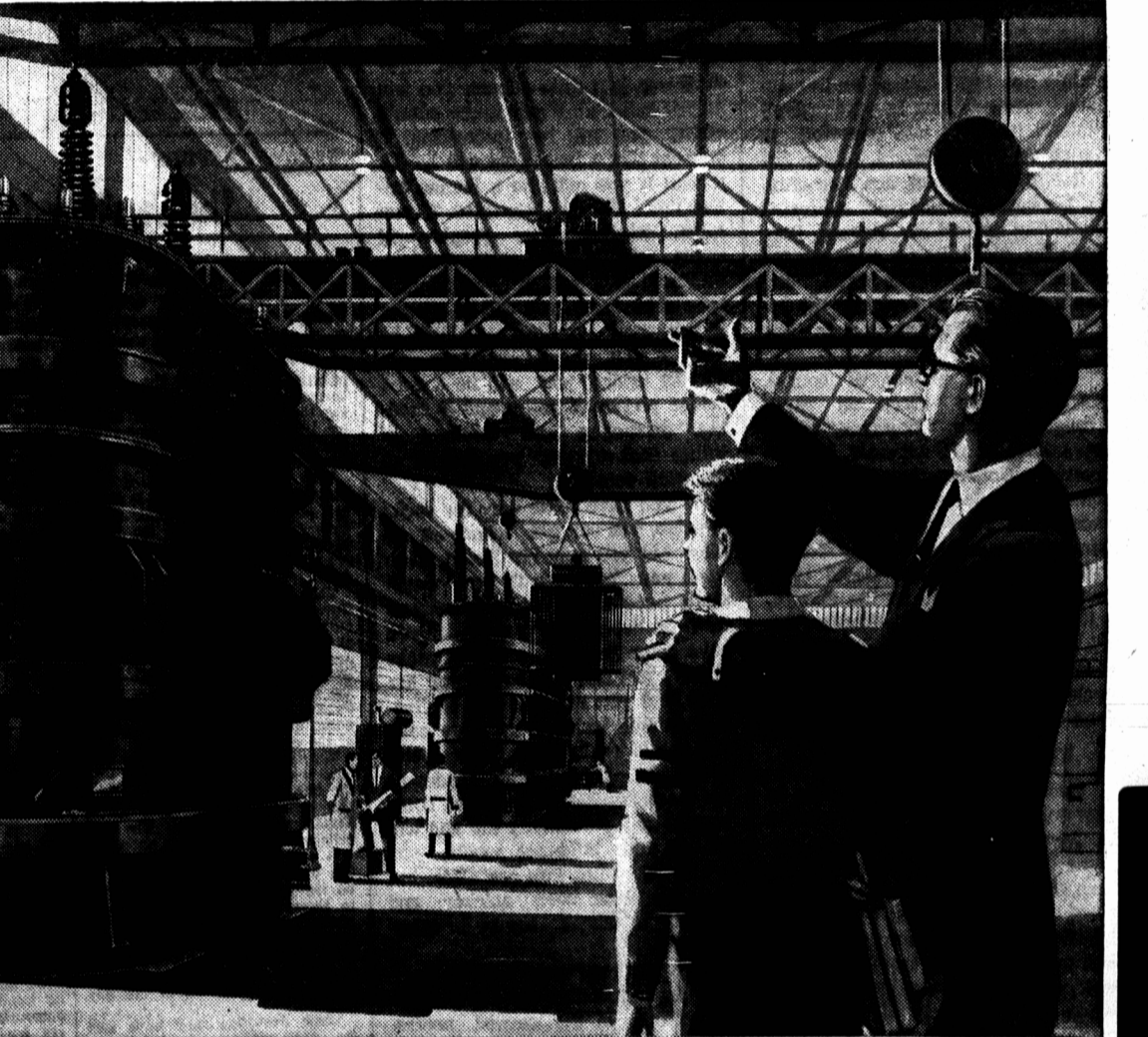
A scene in the Company's new Works at Guelph, Ontario... the largest power transformer plant in Canada. Here, transformers are built for the country's great electric power projects. Many thousands of mathematical calculations are involved in designing transformers, and the wide variety of other electrical equipment manufactured at Canadian General Electric's fifteen plants.
