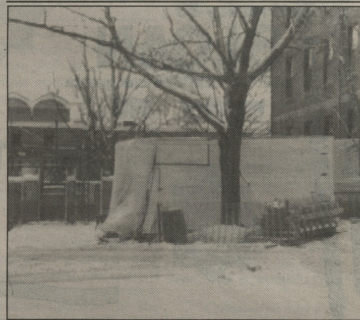
Construction underway at Cass Building.
