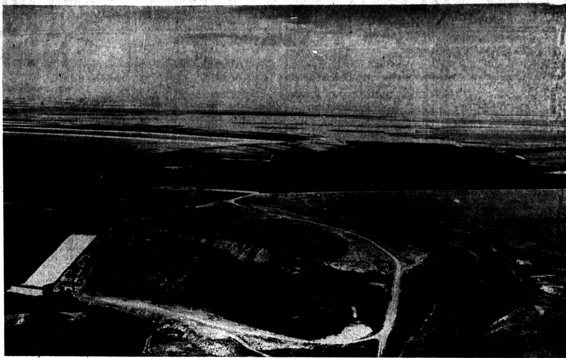
This massive barrier, holding back waters of the St. Mary river in southwestern Alberta, is Canada's largest earth-fill dam. The dam, 200 feet above the normal level of the glacier-fed river, holds water for irrigating 510,000 acres of once-arid land. Just below the giant spillway at left can be seen the outlet from which water flows before entering the main irrigation canal. The St. Mary Milk Rivers Development, of which the dam is part, will cost $60,000,000 before it is completed in 1960. The misty mountains in background of this Alberta government photo are part of the Rockies.—(CP Photo).
