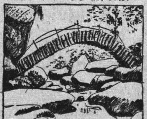
AN ARCHED BRIDGE in the Calnegga Valley, Switzerland HAS BEEN STANDING FOR CENTURIES ALTHOUGH ITS STONES WERE PUT IN PLACE WITHOUT THE USE OF MORTAR
