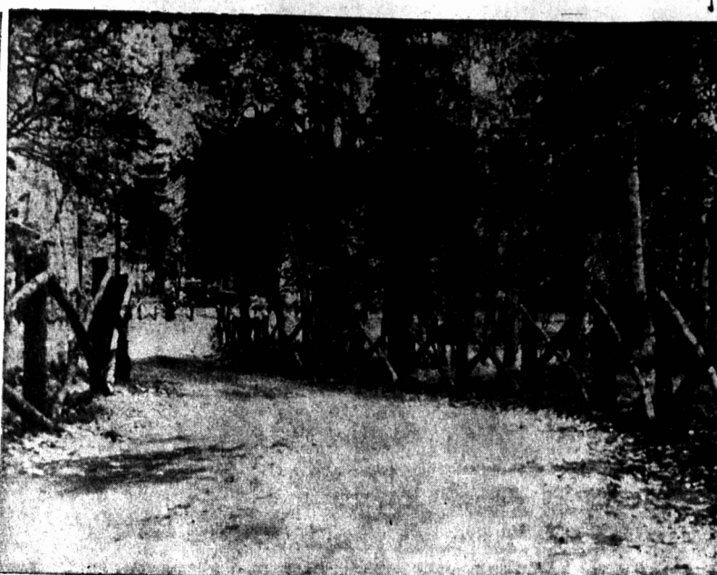
NEW ROADWAY IN VICTORIA PARK
