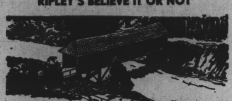
THE ROCKING BRIDGE over the Hovon River, Subarctic and WAS DESIGNED TO SHAKE TO AND FRO THROUGH ANY WINDS OVER IT
