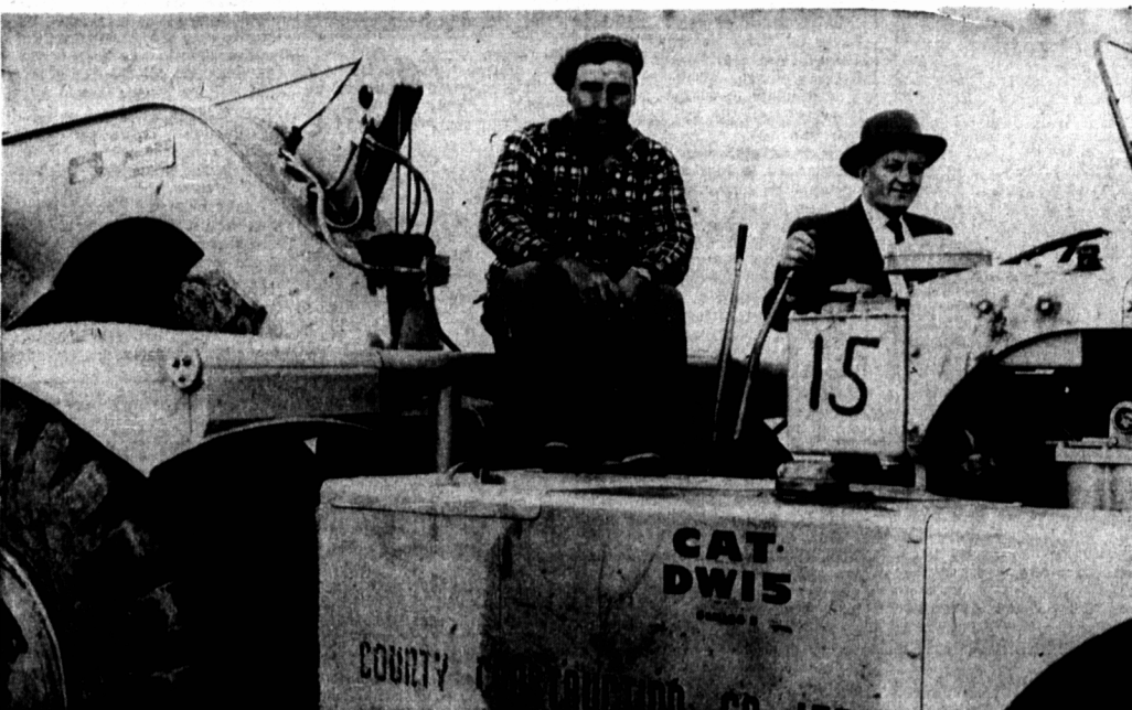
HON. George MacKay is at the controls of the big DW15, earth mover, that hauls the first load for the fill on the Hillsboro Causeway or Western approach to the new Hillsboro bridge. Sitting on top of the big vehicle is George Arsenault, the regular operator.
