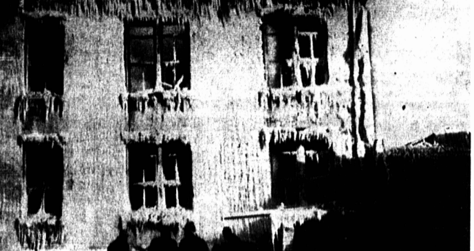
Seen above directing a stream of water through a basement window on the south side of the Summerside Town Hall firemen remained on duty throughout the day and last evening at the ruins of the Town Hall which was completely gutted in an early morning fire. On the top floor, the windows left and center were located in the chambers of the Town Council while the two below these were in the town magistrate's court room. This room was also used by several groups as an assembly meeting hall. The windows (top right) were in the Mayor's office while the police office was directly beneath it. The one storey building which adjoins the main building was used to house the fire department trucks. (Photo by Wotton).
