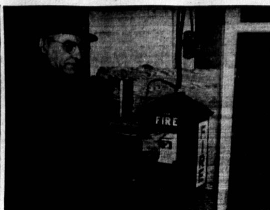
...SUMMERSIDE FIRE Chief Abdom Arsenault presses a button on the control box in the Summerside Fire Hall, to activate a new air horn fire alarm system which was tested yesterday. Photo by Wotton
