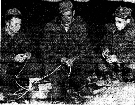
Three members of the RCE, prepare a charge of dynamite to open a new gravel pit for road construction in Korea. Left to right: Cpl. E. V. Marks, Charlotte St., Sackville, N.B.; Spr. J. W. Mercer, 12037—88th St., Edmonton, Alta.; and Spr. C. J. Dockendorff, 23 Orlebar St., Charlottetown, P.E.I.
