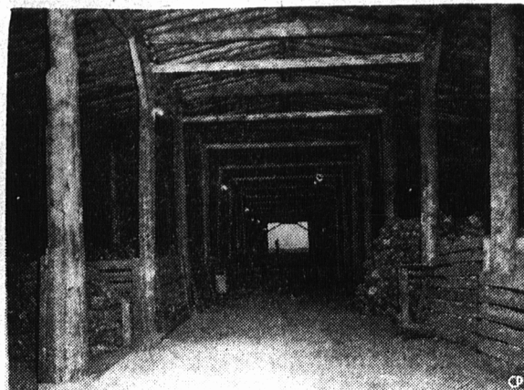
HUGE ROOT CELLAR—Believed to be the biggest in Canada, this root cellar at Lethbridge, Alta., has a storage capacity of 200 train carloads of vegetables. Storage for turnips and potatoes is in bins with 62-foot-long loading ways beside each. This root cellar is 235 feet long and 125 feet wide and can hold 80 semi-trailers at the same time, with the central driveway still left clear. (CP Photo).
