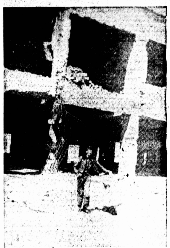
April, 1951. Another view of bombed administration building, with S/Sgt. Davis in foreground.
