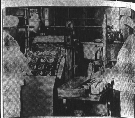
All bottles are passed through several processes and thoroughly sterilized. Then they are automatically filled and sealed.
