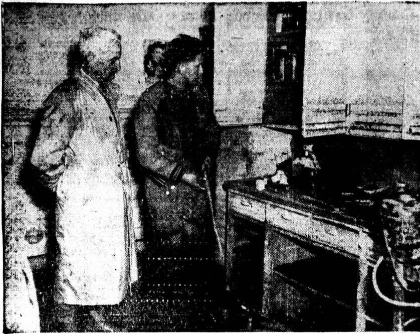
Desolation and destruction and a high-water mark etched in slime in the ruined kitchen of the home of H. J. Murray, Storekeeper of Morris, Manitoba, which bore the full brunt of the flood waters of the Red. Here, Major General Harold J. Riley, Chairman of the Restoration Committee of the Manitoba Flood Relief Fund surveys the wreckage with Mr. Murray's son, Jack, a first-year medical student. Scenes like these are duplicated in thousands of homes throughout Southern Manitoba and Winnipeg. It is to relieve at least a measure of the personal loss that the Manitoba Flood Relief Fund continues its plea for funds. Send your contribution direct to Fund Headquarters in Winnipeg, or to any Chartered bank in Canada. Your donation will be tax exempt.
