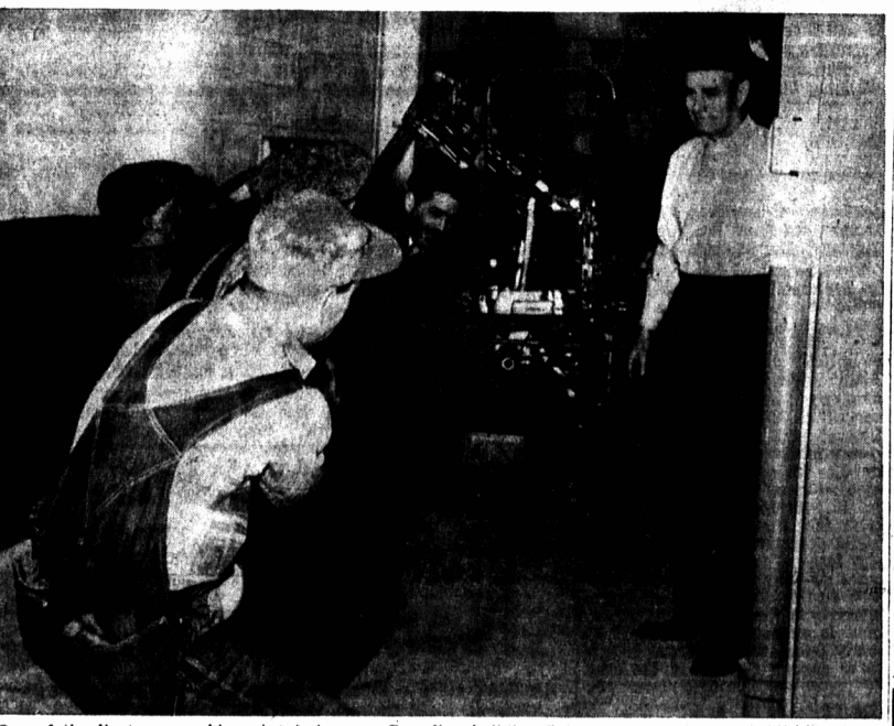
One of the linotype machines is being landed on the second floor of the new Guardian building Saturday morning. Mr. Ben Floyd (right), supervises the placing of the machine.
