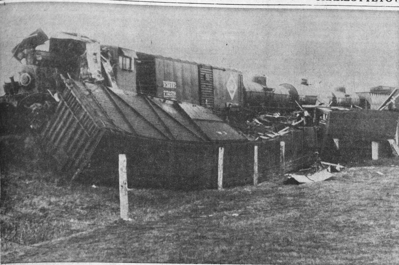
THE DAMAGED engine of the mixed passenger and freight train can be seen behind the overturned and badly damaged box car at the train collision scene west of Travellers Rest crossing. In the right foreground is the wreckage of the caboose from the freight train.
