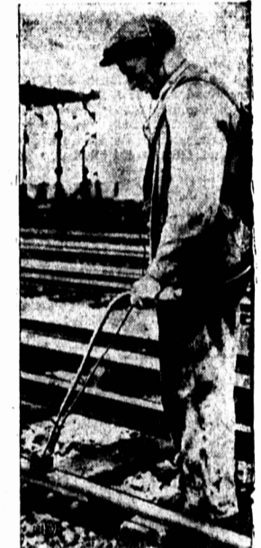
"Audiogage" is an instrument to detect flaws in r.r. tracks.
