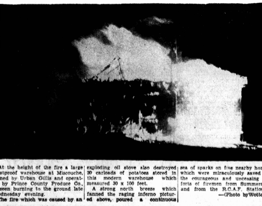
At the height of the fire a large frostproof warehouse at Miscouche, owned by Urban Gillis and operated by Prince County Produce Co., is seen burning to the ground late Wednesday evening. The fire which was caused by an exploding oil stove also destroyed several carloads of potatoes stored in this modern warehouse which measured 30 x 100 feet. A strong north breeze which fanned the raging inferno pictured above, poured a continuous sea of sparks on five nearby homes which were miraculously saved by the courageous and unceasing efforts of firemen from Summerside and from the R.C.A.F. Station. —(Photo by Wotton).
