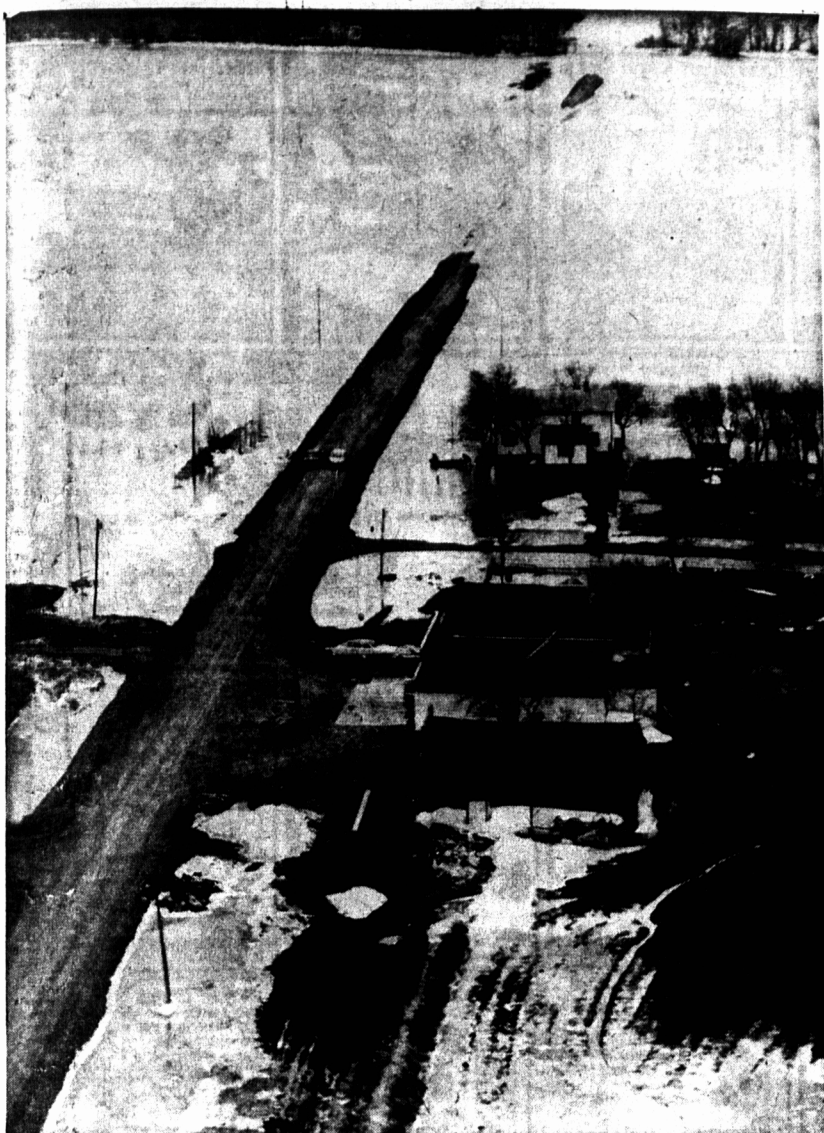
FLOOD CUTS HIGHWAY
