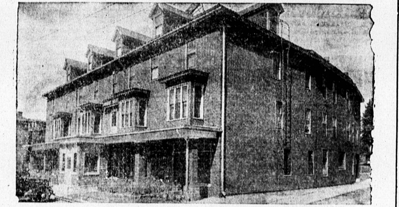
The Amberst Hotel at Amherst, N. S., after the application of Brantford Insulated Siding
