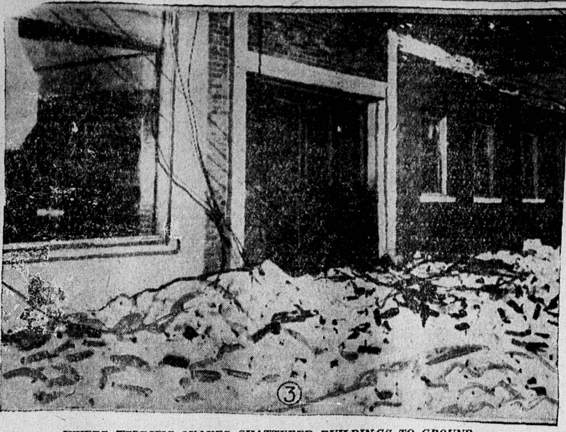
WHERE TERRIFIC QUAKES SHATTERED BUILDINGS TO GROUND Here is a general scene of wreckage in the quake area of southern California where over a hundred are dead and thousands injured as the state and country moved to put the area under martial law and provide immediate relief.
