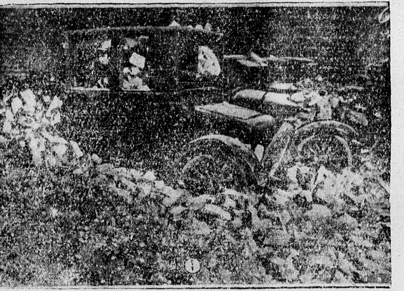
WALLS OF GARAGE CRASH UPON CARS The above picture gives a slight idea of the terrific force of the shocks in the earthquake area of southern California. The ruins of the car shown above were caused when the tremors shook the walls of the garage around it.
