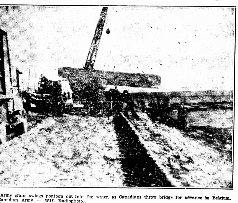
Army crane swings pontoon out into the water, as Canadians throw bridge for advance in Belgium. (Canadian Army - WIE Radiophoto)
