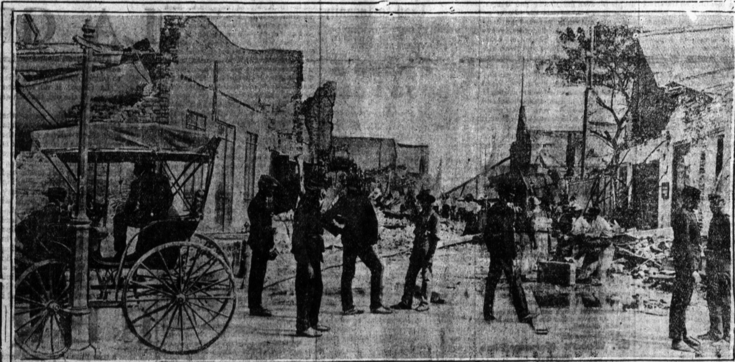
Every House On Harbor Street Was Destroyed
