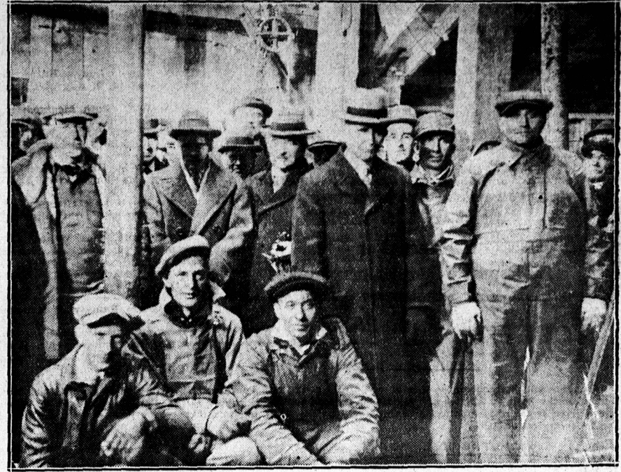
This picture was taken just before Premier Stewart turned on the steam which started the drilling for oil on Governor's Island, December 1st, 1925. From left to right standing may be seen R. M. Stuntz, Field Manager for Henry L. Doherty Company. He is standing alongside the solid steel drill stem which is 32 feet long and weighs 2400 lbs., on which is screwed on the ponderous bit 24 inches in diameter, 6 feet long, and also weighing 2400 pounds, which is ready to begin its downward course in search of oil. Mr. R. H. Jenkins, M. P., is standing just behind the drill; next to him is Mr. E. M. Gunsaulus, United States Consul, Judge Stewart, and Chief Justice Matheson, Premier Stewart is next to the Chief Justice, and the others are Mr. J. A. MacDonald, M. P., W. M. Murphy, driller, C. H. Harter (in overalls) driller, and Mr. H. H. Shaw. Sitting left to right are B. R. E. Polnsett, office manager for the Doherty Company, C. C. Bonley, tool dresser, and George M. Perkins, tool dresser.
