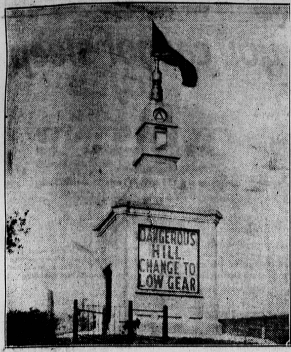
A HIGHWAY "LIGHTHOUSE" FOR SAFER TRAVELLING This novel method of warning motorists of their approach to dangerous curves or hills has been adopted in England. The first "lighthouse" is located at a dangerous place on the road between Manchester and the Potteries. The use of lights as a warning is not new in Canada, but this land "lighthouse" throws a beam of light which is visible several miles away.
