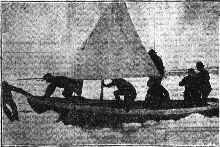
Crossing at the Capes.
