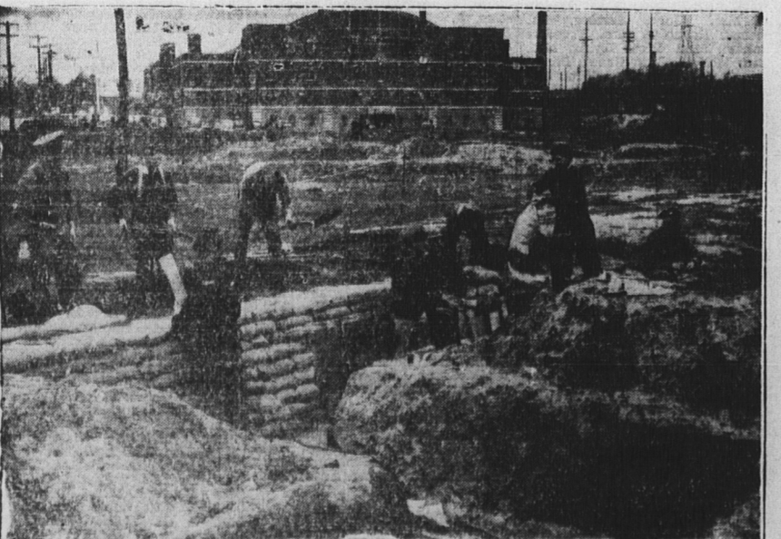
From swinging pick and shovel with R.C.E. recruits at Toronto, Then the Ontario minister of public works went to Gibraltar, to command a tunnelling company of engineers. They're all hard-rock miners in the company now drilling under the rock at Gibraltar, but
